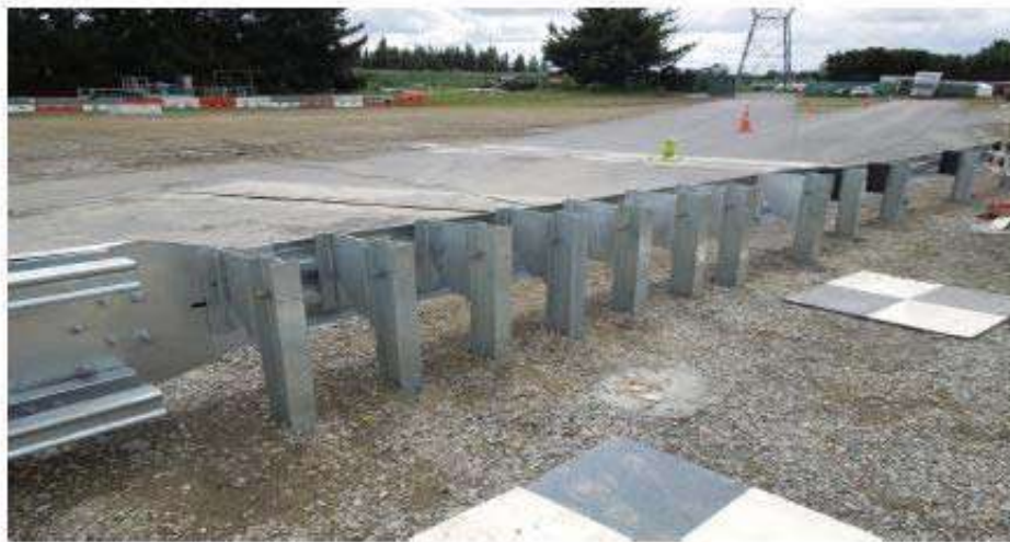
Transition from Roller Barrier to Thrie Beam
